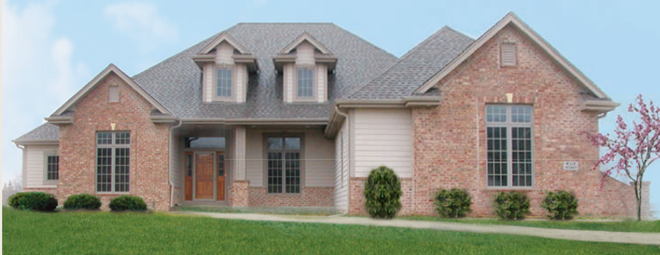
Shown with optional brick light pier off garage.
